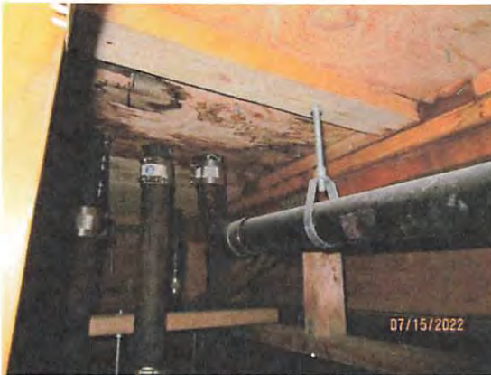
Photo 23: Underside of men's shower area
