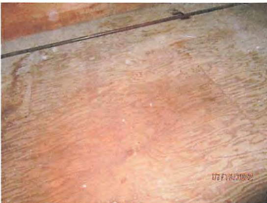
Photo 25: Interior soffit sheathing under men's lockers
