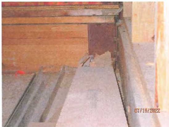
Photo 31: Grid C2 framing - flash on
