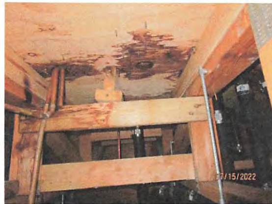
Photo 24: Underside of men's shower area
