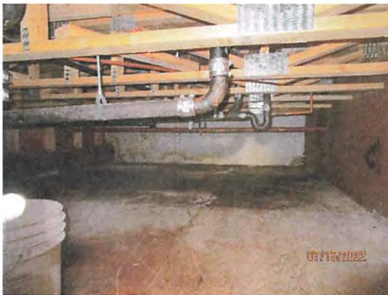
Photo 12: Crawlspace area under women's shower & sauna
