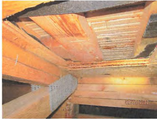
Photo 7: Ball court flooring construction
