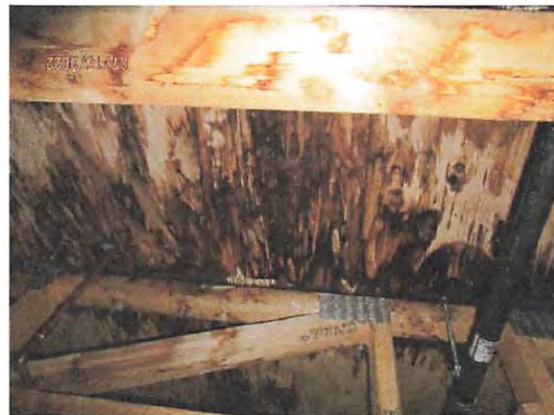
Photo 13: Underside of sub-floor at women's sauna
