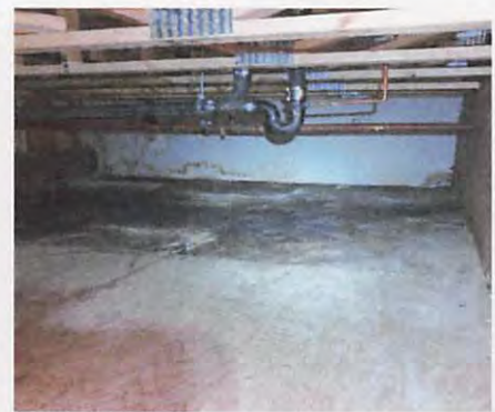
Photo 3. Beneath women's sauna.
